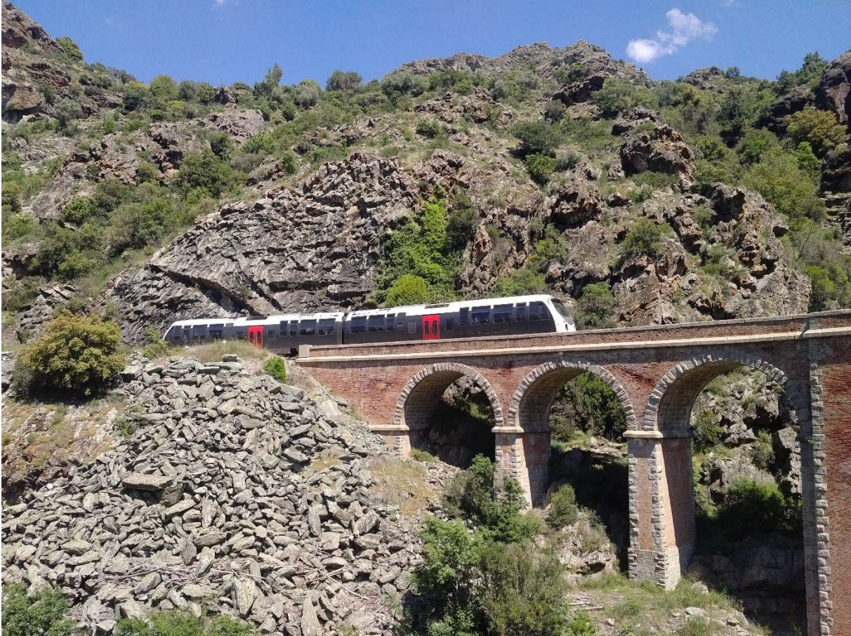
Train AMG800, on the Ponte Novu bridge.
