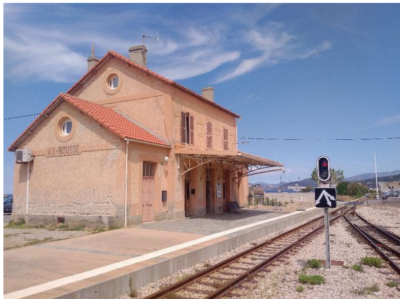
Ile Rousse station, with the simplified signal system, a unique signal used for 3 tracks
